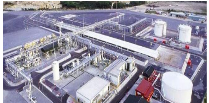
( Nam Con Son Gas Pipeline Facility - Vũng Tàu Factory )
